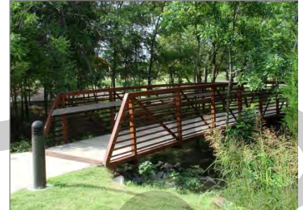
Bridge at Shores Park 2024: A pedestrian bridge connecting two (2) play areas and extending over a riparian area at Shores Park.
